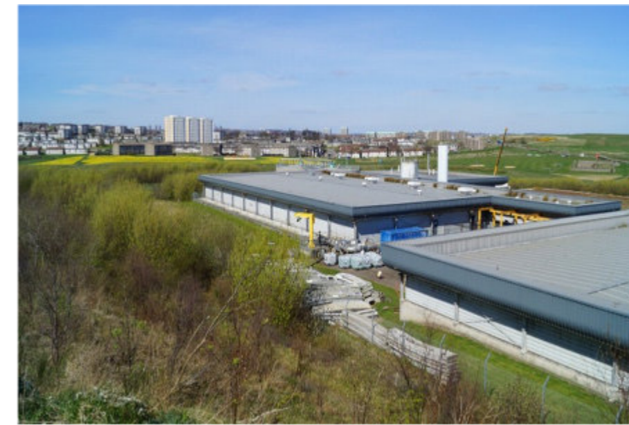
Nigg Waste Water Treatment Works
